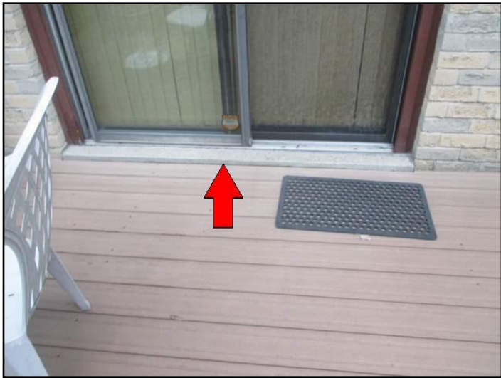
Threshold - clearance inadequate (above...
