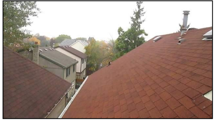
The roof covering appears to be within the...
