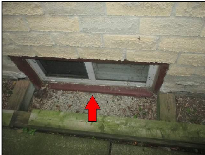
Window Well - clearance inadequate below...
