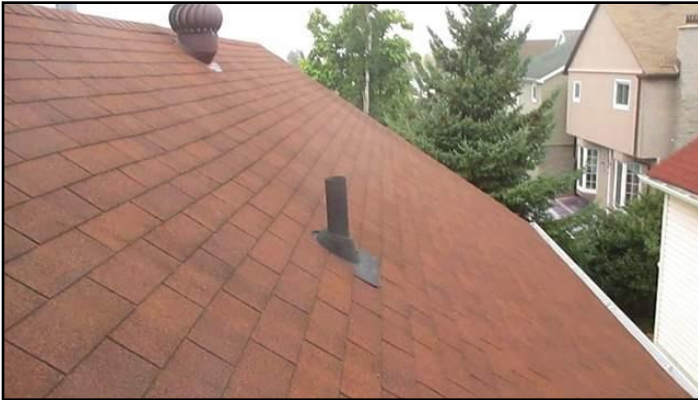
The roof covering appears to be within the...
