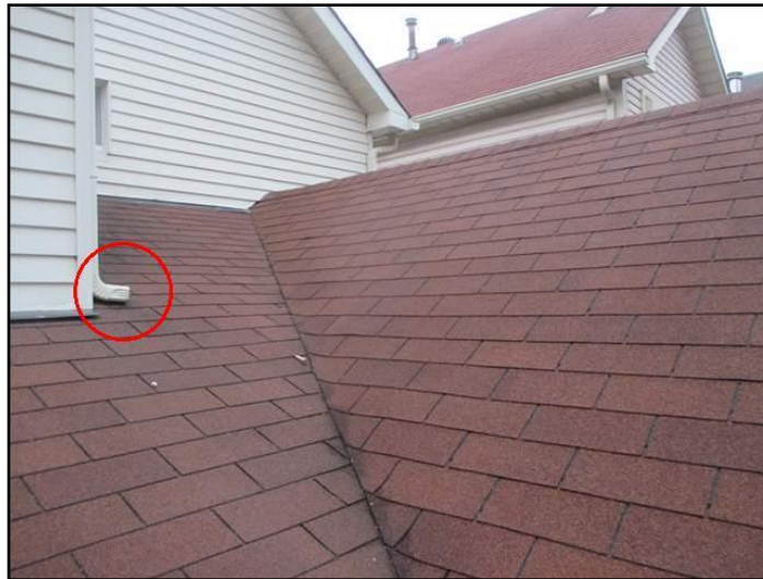
Discharge onto lower roof (causes premature...
