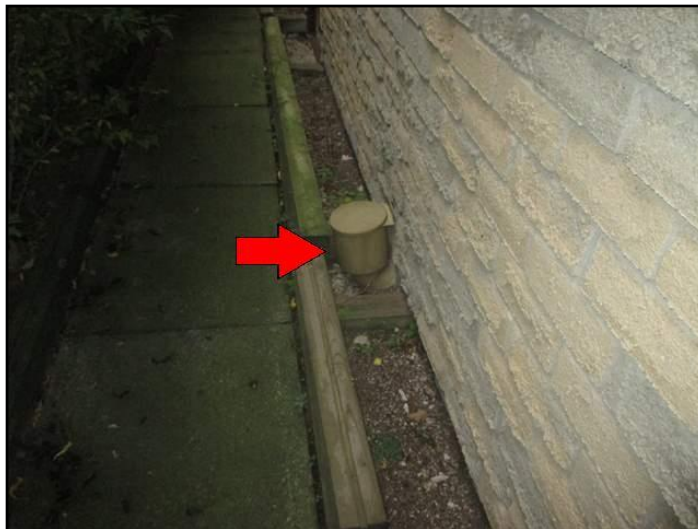
Vent too close to grade
