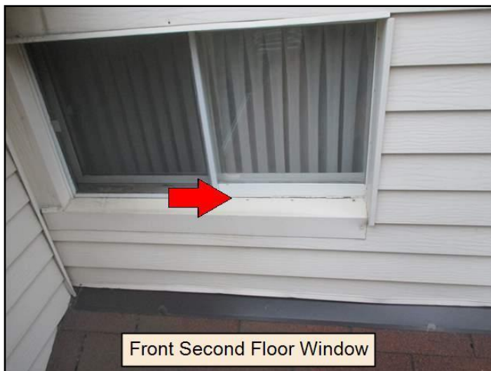
Example: Caulking - deteriorated or missing
