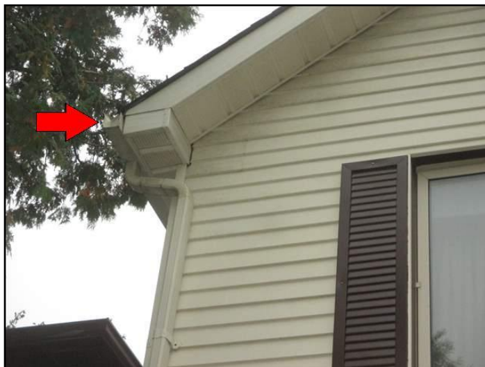
End cap damage
